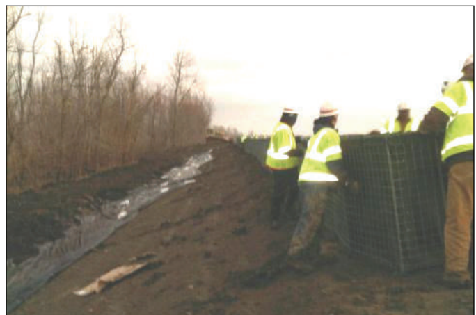
Crews install HESCO barriers at the upper crevasse Wednesday evening.
