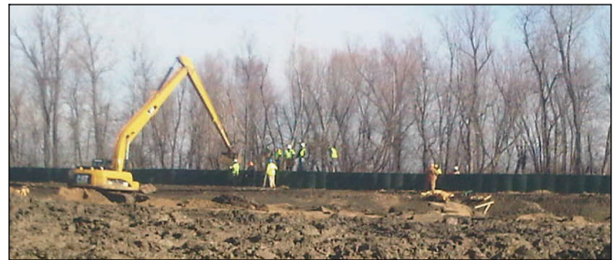
A crew fills HESCO barriers at the upper crevasse Friday. The barriers are a temporary measure to raise the level of protection at Birds Point from 51 to 55 feet on the Cairo gage. Permanent repairs to the levee will resume after spring highwater recedes.
